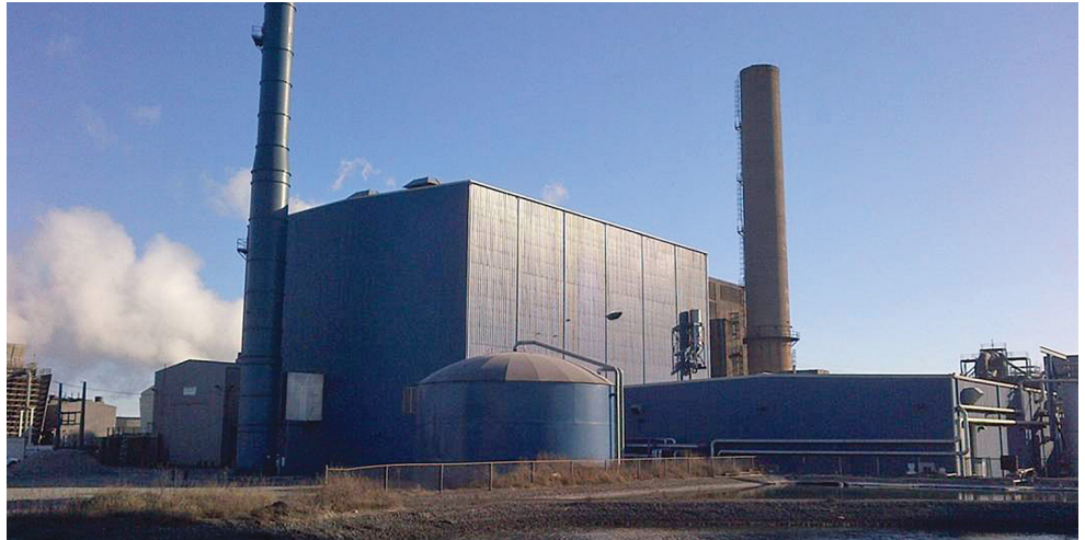
Combined heat and power system at ArcelorMittal's Indiana Harbor steelmaking facility in east Chicago.
